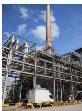
Gas Turbine 1 Stack
